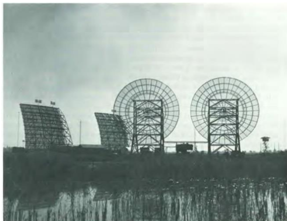
The Phu Lam BACKPORCH Site
